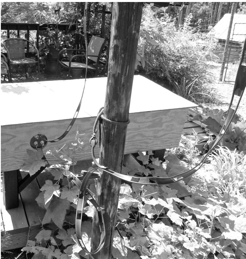
Photo A — Here is the antenna feed point. The ladder line from the shack (not visible in this photo) comes to the pole from the left, then down to the tuner box. The coax and control cables are fed through buried electrical conduit. You can see a corner of my outdoor patio, where the tuner box serves as a convenient summer serving table.
